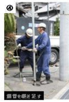
⑤ 鋼管を掘り出す
