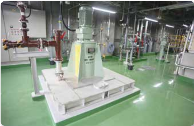
Nitrification tank mixer and reaeration equipment
