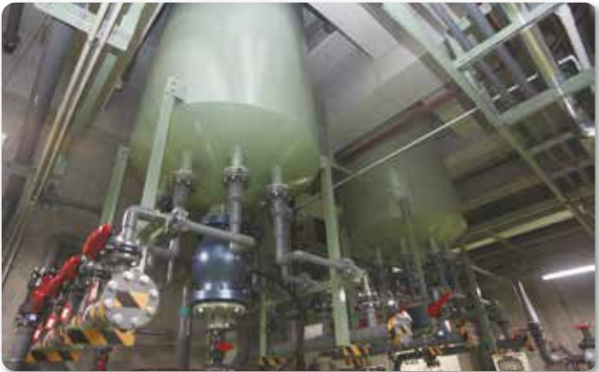
Activated carbon adsorption equipment
